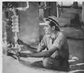
A Fls. 400 supplemental award goes to W. de Souza for his idea which has already won an initial Fls. 100 and a capital Fls. 400. His idea was to install a sight glass in catalyst loading line from 1/2 ton hopper.
